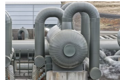
• the water supply pump station
